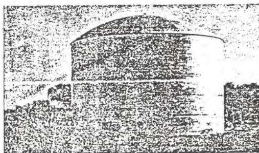
Figure —Umbrella-Roof Tank
