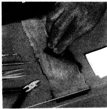
1. Roughening of the application area
